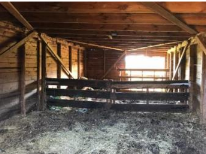
BG2 sealed eaves, single skin wood roof
