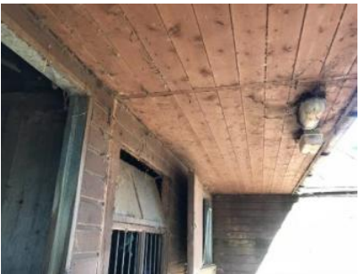
Showing sealed eaves BG3
