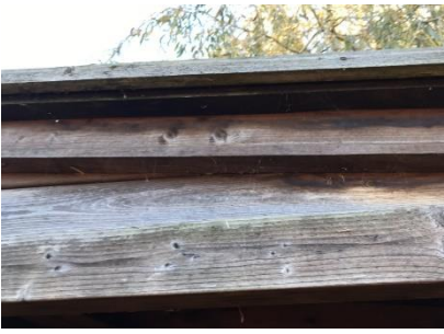
Showing sealed eaves BG3
