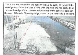
This slide shows the rough edge of the concrete base covering the rear of the pool, 11-06-2015. The shingle /sand placed by the Council has been washed away by the tide. This rough edge has cut and grazed the feet of many children. It is my contention that the QLM inspector did not see the true day to day nature of the base of the pool.
