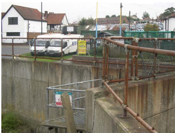
Fig. 35 Ferry Road, concrete revetment around the sluice at the end of the creek
