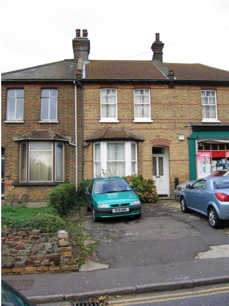
Fig. 8 No. 103 High Street, a well preserved Victorian cottage typical of the late 19th-century development at the southern end of the village in the vicinity of the station. Brickwork and windows are intact but it has lost its slate roof.
