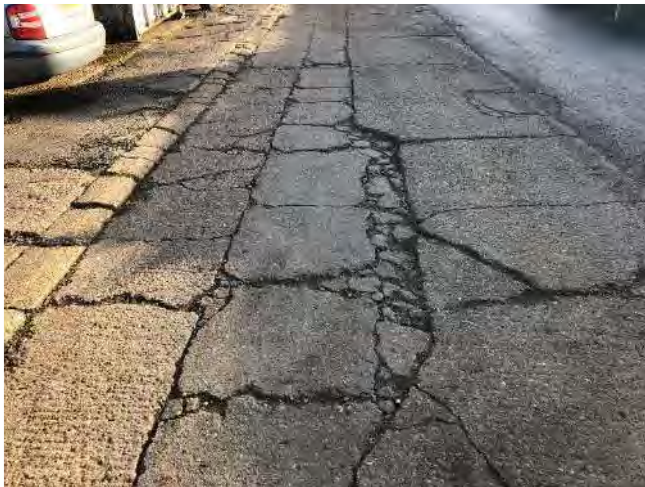
Plate 1: Elongated pot hole up to 50mm deep
