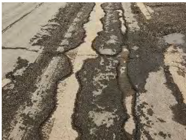
Plate 32: Flexible overlay deteriorating
