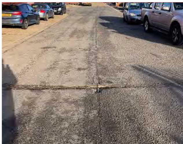
Plate 9: Flexible overlay cracking at joints
