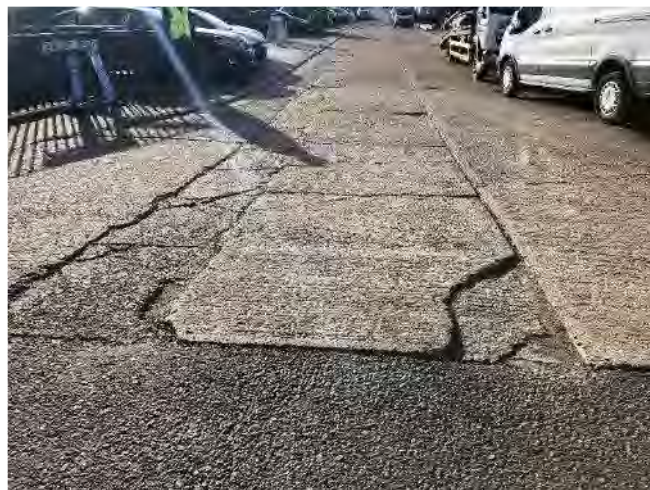
Plate 5: Potholes and cracked surface
