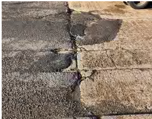
Plate 8: Flexible overlay lifting from concrete surface below
