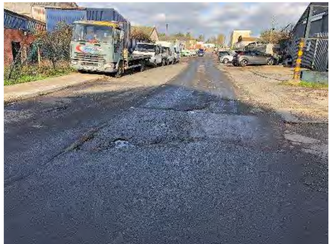
Plate 19: Road surface deteriorating
