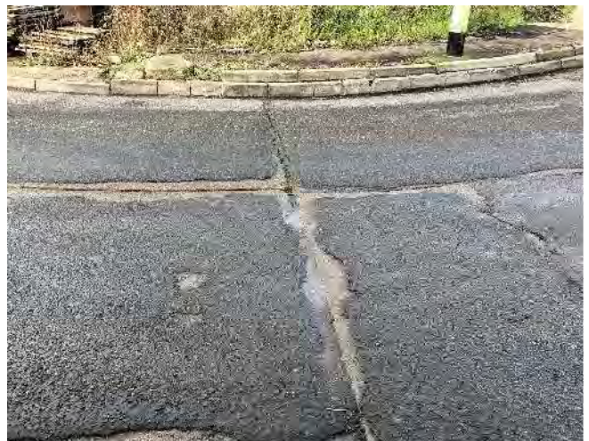
Plate 21: Exposed joints
