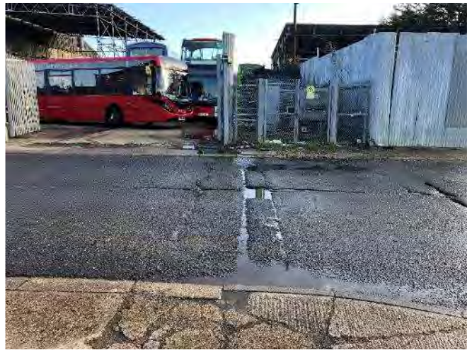
Plate 13: Run off from adjacent site
