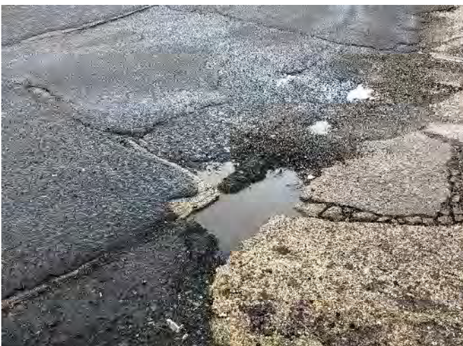
Plate 20: Potholes on carriageway edge
