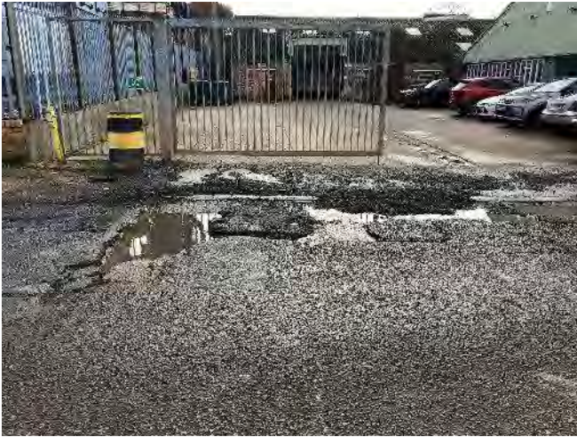
Plate 24: Eroded tarmac
