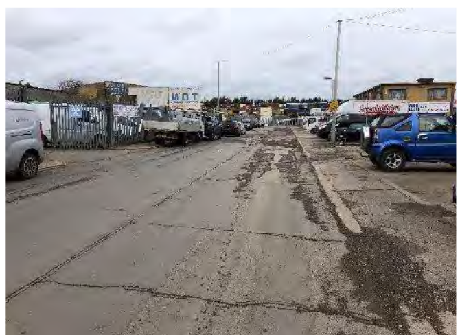
Plate 33: Reflective cracking of surface
