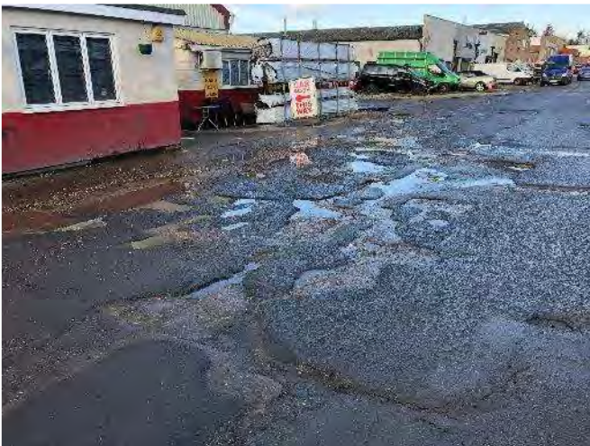
Plate 18: Potholes and surface cracking
