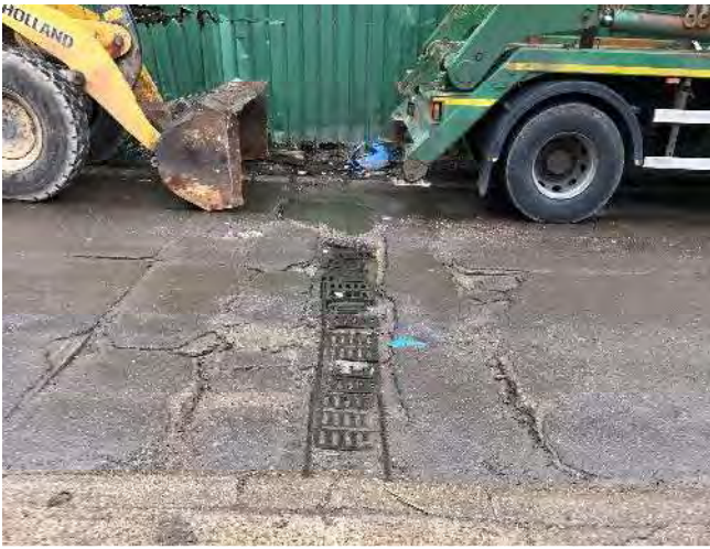
Plate 51: Concrete around drain cracking
