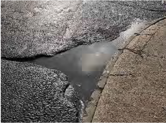
Plate 16: Water pooling at blocked gulley
