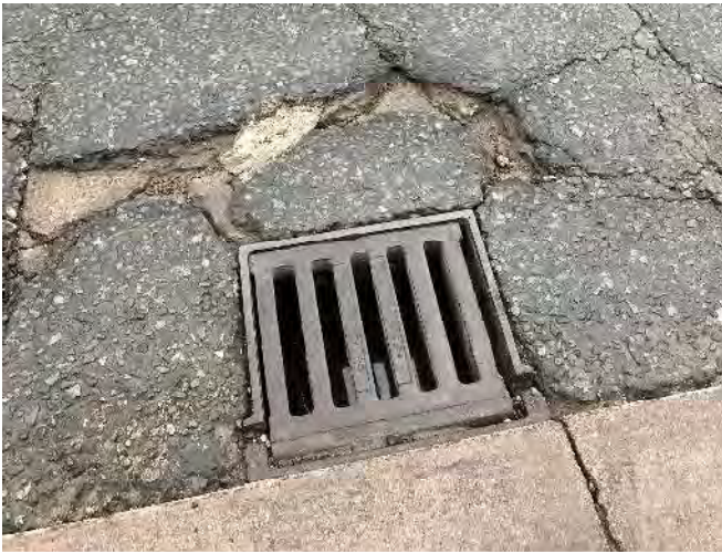
Plate 40: Surface deterioration around gulley
