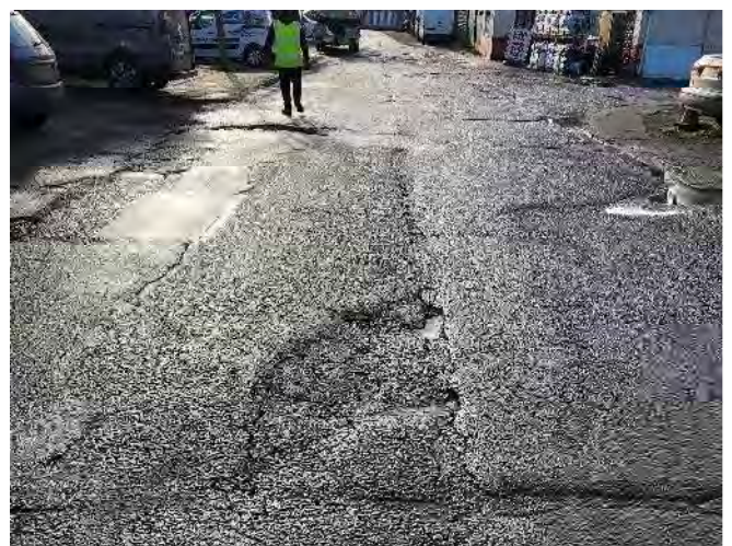
Plate 15: Potholes up to 80mm deep
