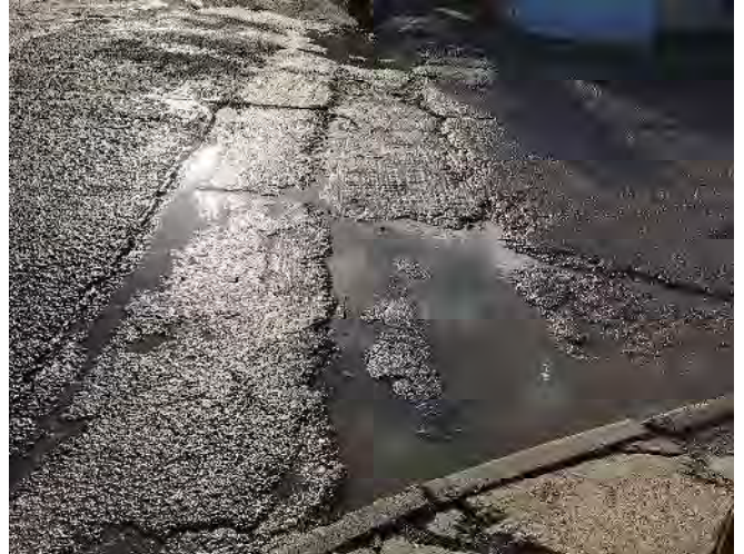
Plate 17: Potholes up to 80mm deep
