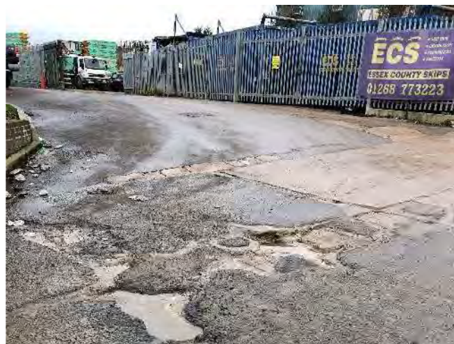
Plate 44: Potholes and cracks
