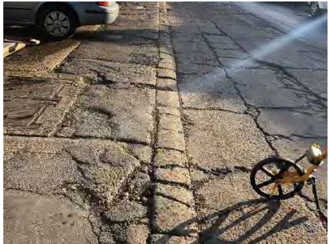
Plate 2: Damaged footway & broken Kerbs
