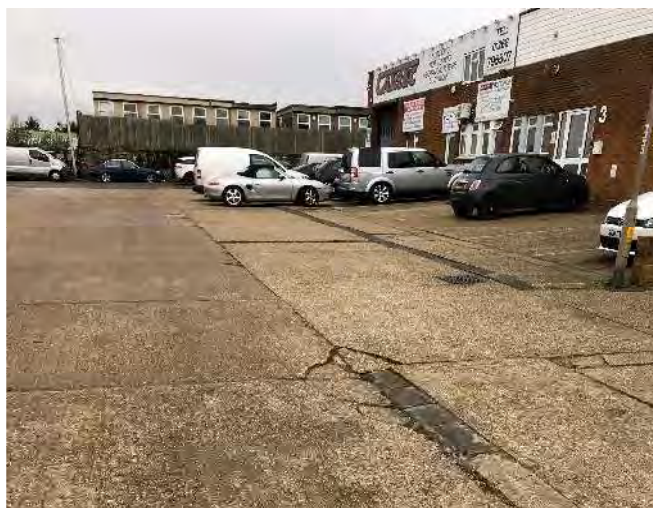
Plate 47: Cracks on carriageway edge
