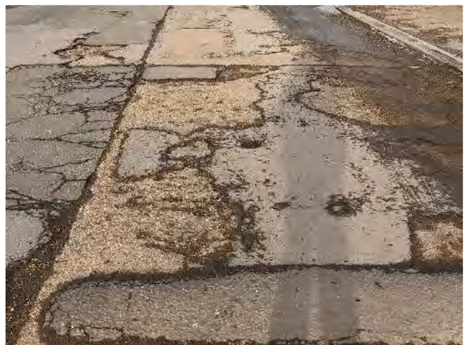
Plate 27: Uneven surfacing
