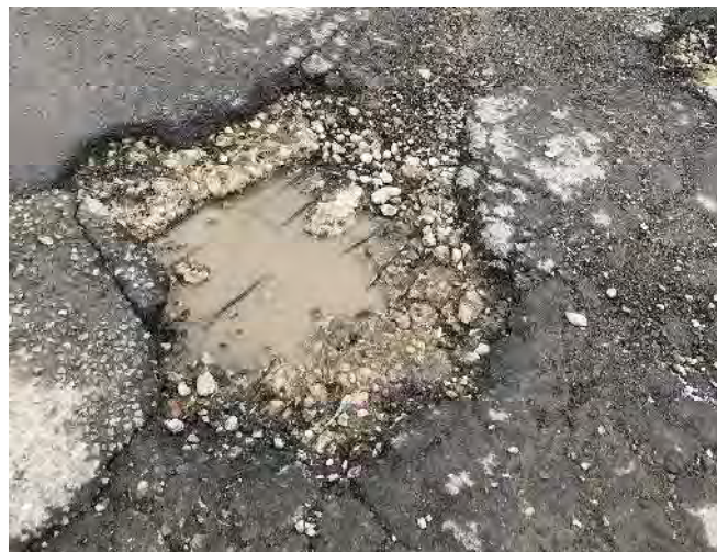
Plate 36: Steel bars exposed in pothole
