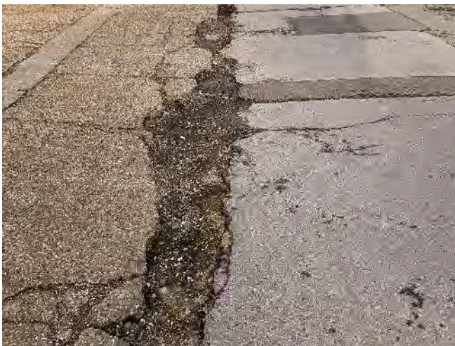
Plate 26: Carriageway edge deteriorating
