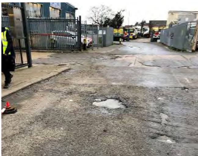
Plate 49: Potholes in carriageway
