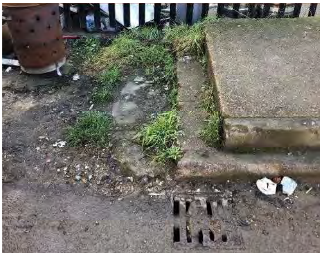
Plate 3: Blocked gulley
