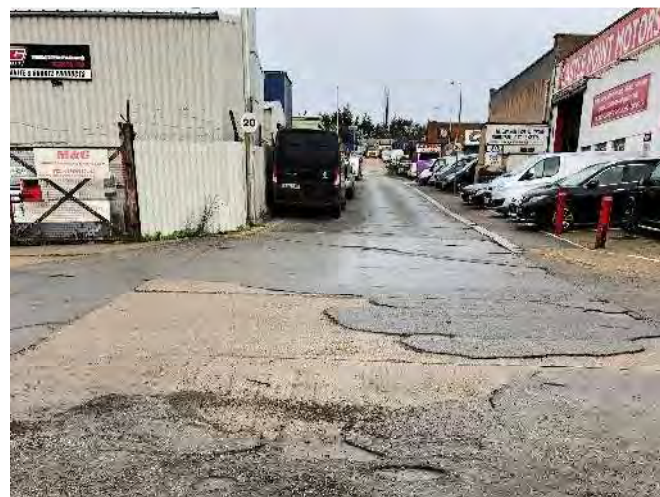
Plate 38: Overlay lifting at junction
