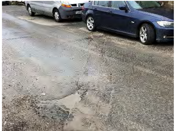
Plate 43: Service trench deteriorating
