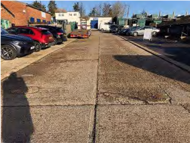
Plate 6: Cracked concrete and surface deterioration
