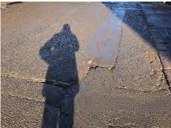
Plate 14: Service trench cracking
