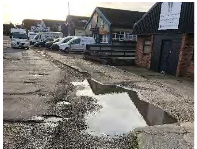
Plate 31: Pothole filled with water
