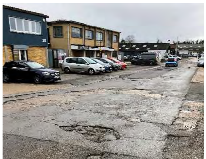
Plate 37: Flexible overlay deteriorating
