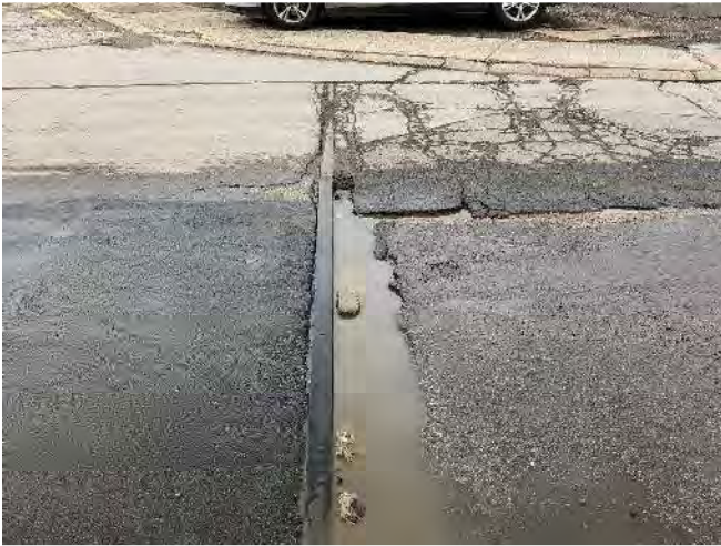
Plate 30: Corner of slab broken
