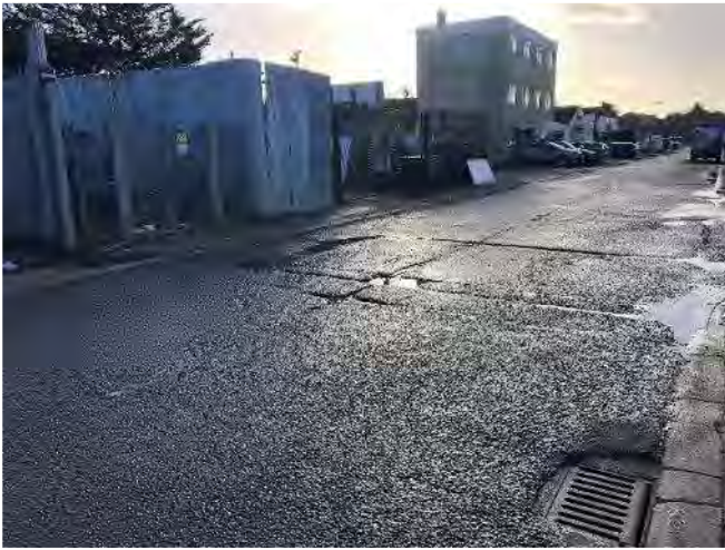
Plate 12: Water pooling at junction
