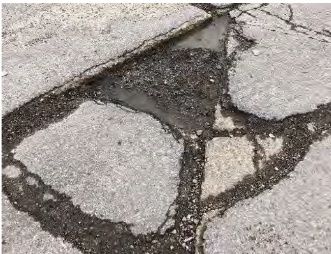
Plate 30: Corner of slab broken
