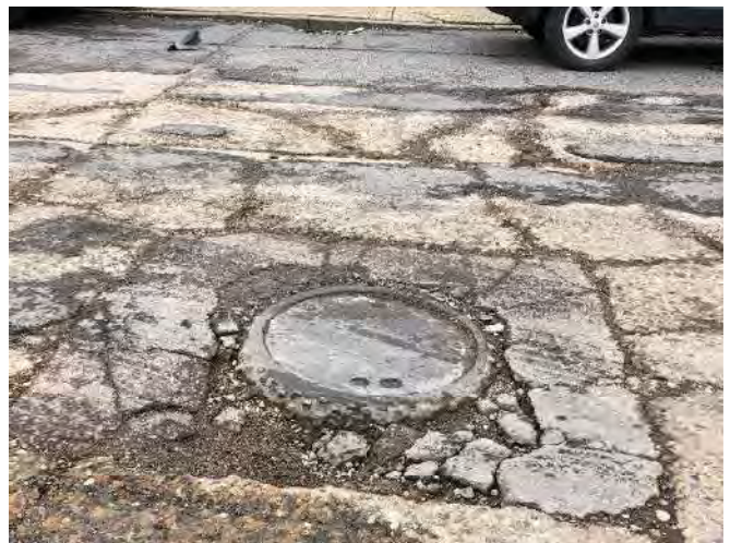
Plate 35: Erosion around manhole cover
