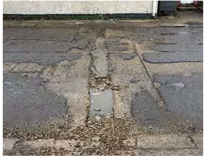
Plate 52: Service trench deteriorated
