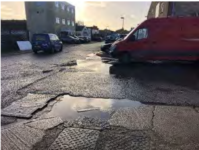
Plate 12: Water pooling at junction
