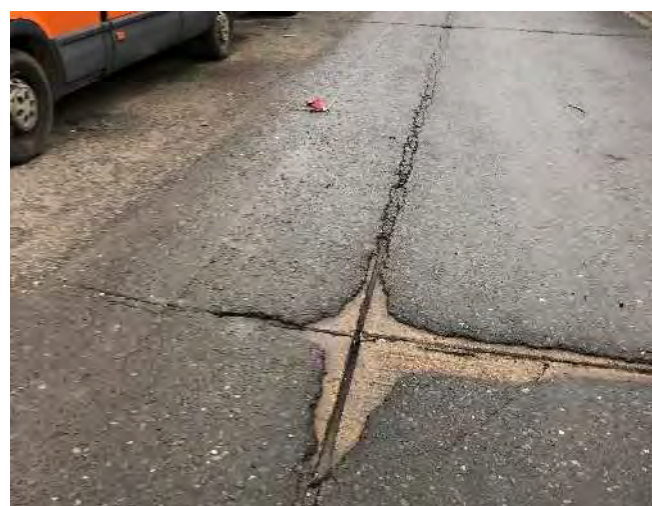
Plate 50: Tarmac cracking at joints
