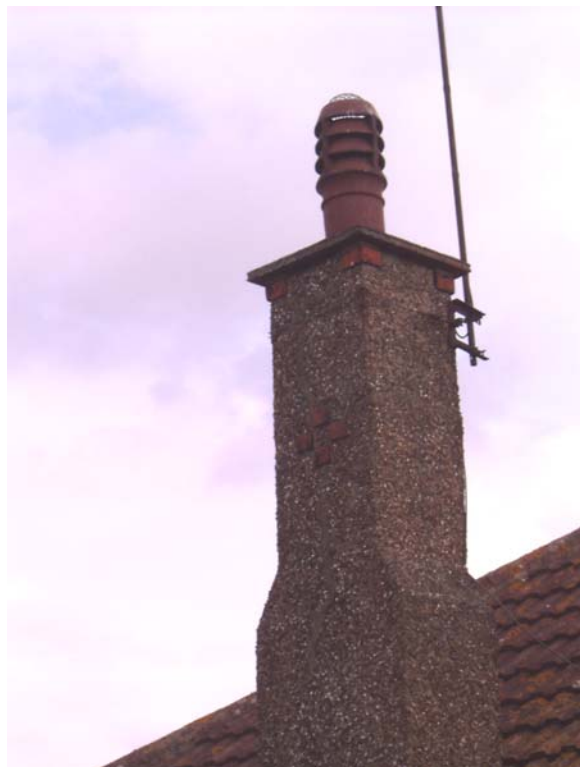
Fig. 7. Chimney stack finished in pebble dash.
