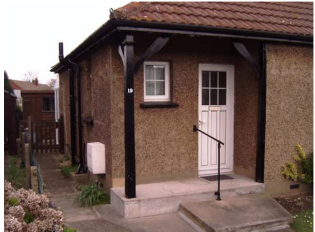
Fig. 11. Recessed front wall to create porch
