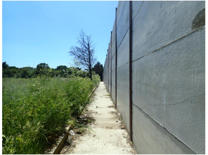
Photograph 2 - Sealed Curbing
